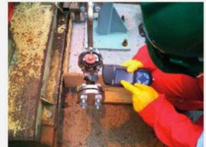
Tagged assets can be instantly scanned and identified using handheld devices
